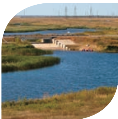
Hydraulic structure of Konchubai Gully
