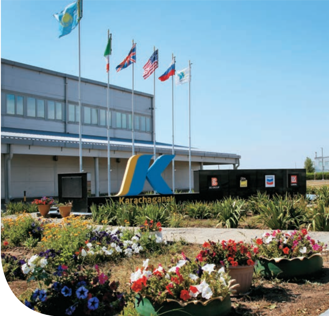
KPC field administrative building
